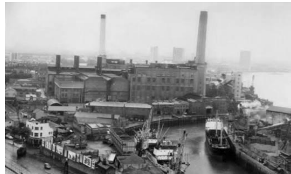
Deptford Power Station on the side of Deptford Creek
